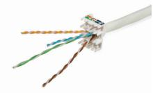
Insert the wires into the cap through the hole.
